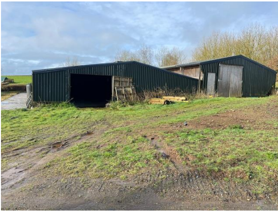
Buildings to south of site
