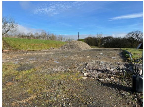
Buildings have now been demolished
