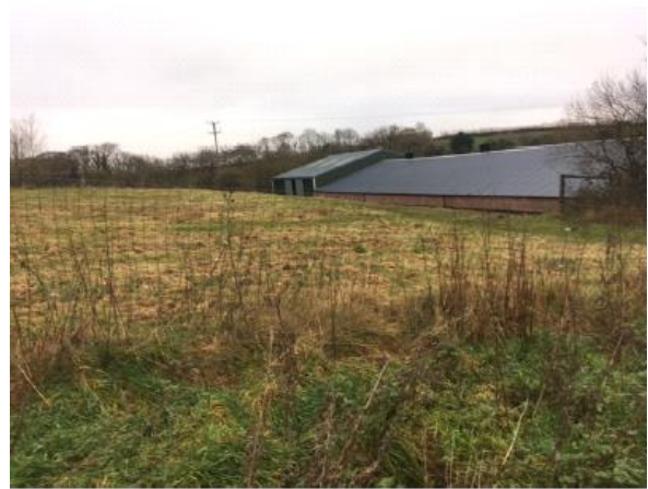
Original buildings when viewed from the west
