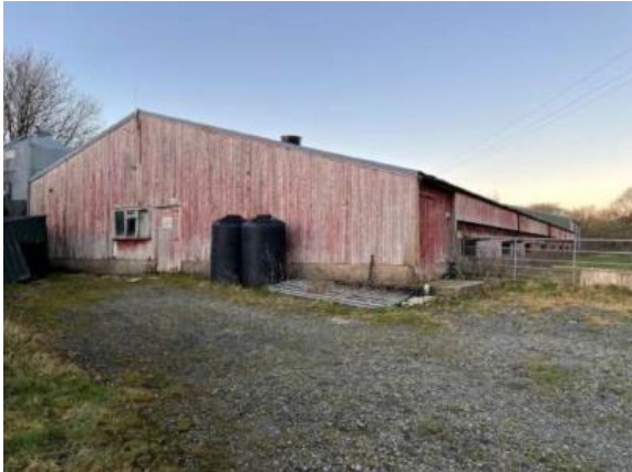
Gable end of original building facing northwards
