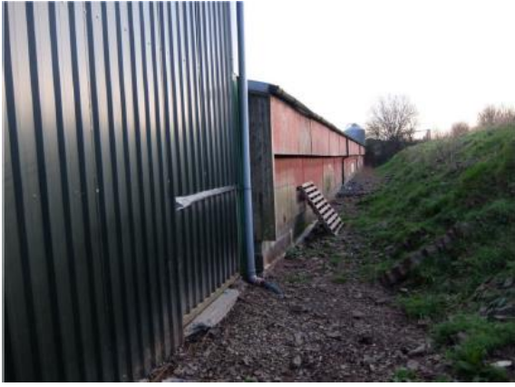
Excavated bank to rear of original buildings
