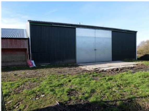
Eastern elevation of taller steel portal framed addition
