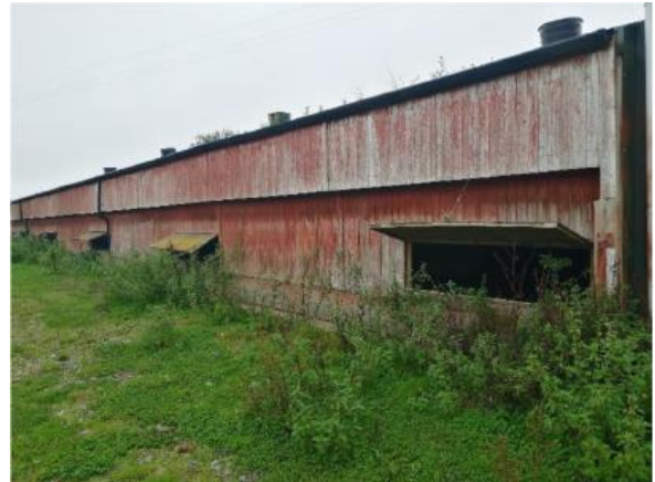
Eastern elevation of original building
